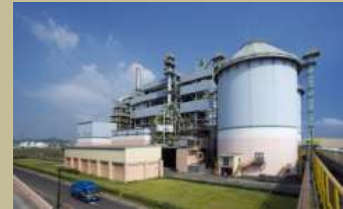
RDF Power Plant
