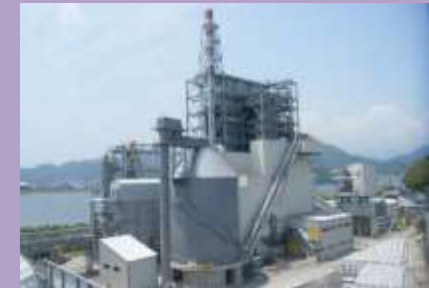
Biomass Power Plant
