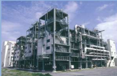
Sewage Sludge Incinerator
