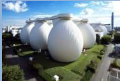
Power Generation using Digestion Gas
