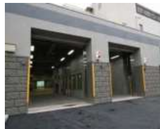
Entrance Weighing Bridge
