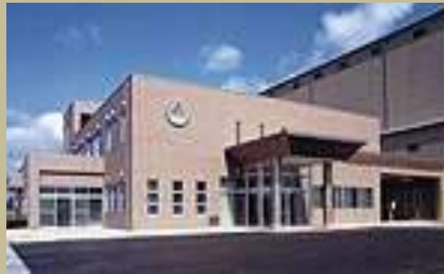
RDF Production Plant
