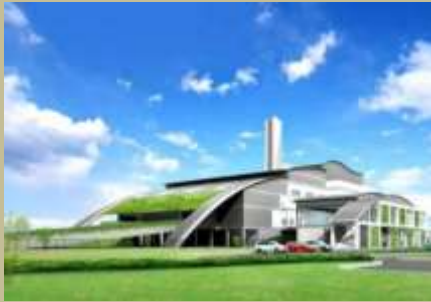
Waste to Energy Plant
